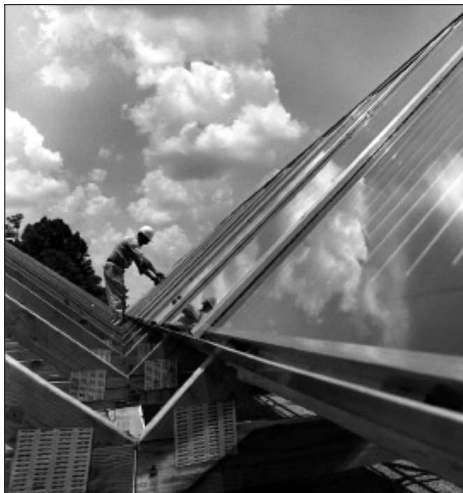
The dedication of the nation's largest solar heating and cooling system then in operation took place November 26, 1975, at the George A. Towns Elementary School in Atlanta, Georgia. Solar collector panels mounted on the roof are pictured during construction. It was expected that the system would supply more than 60 percent of the year-round heating and cooling for the 32,000 square-foot building. A conventional gas-fired boiler supplements the solar system. Credit: ERDA Photo by Frank Hoffman, courtesy AIP Emilio Segrè Visual Archives, Physics Today Collection.
